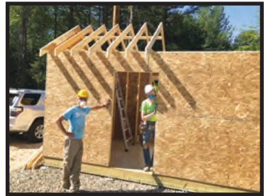
Volunteers at the Shutesbury build site
