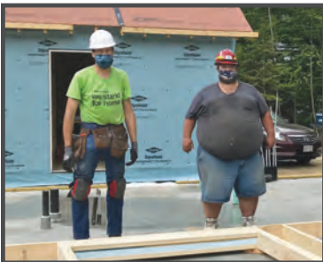
Chuck helps raise the first wall on his future home
