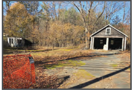
Pelham site with shed
